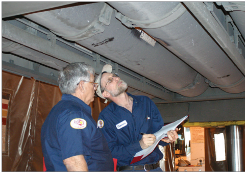
Use the Inspection Form to Document Each Step
