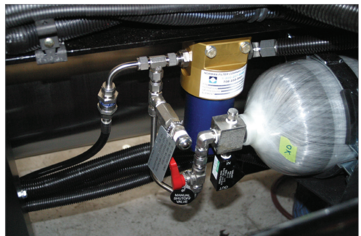
Cylinders and Safety Devices are Designed for the Pressure
